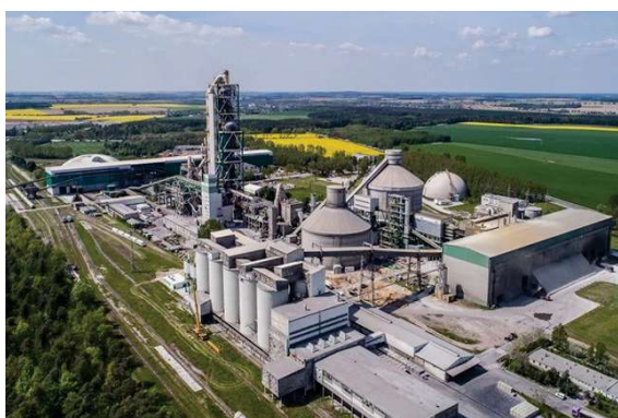
Cementownia Kujawy Holcim
